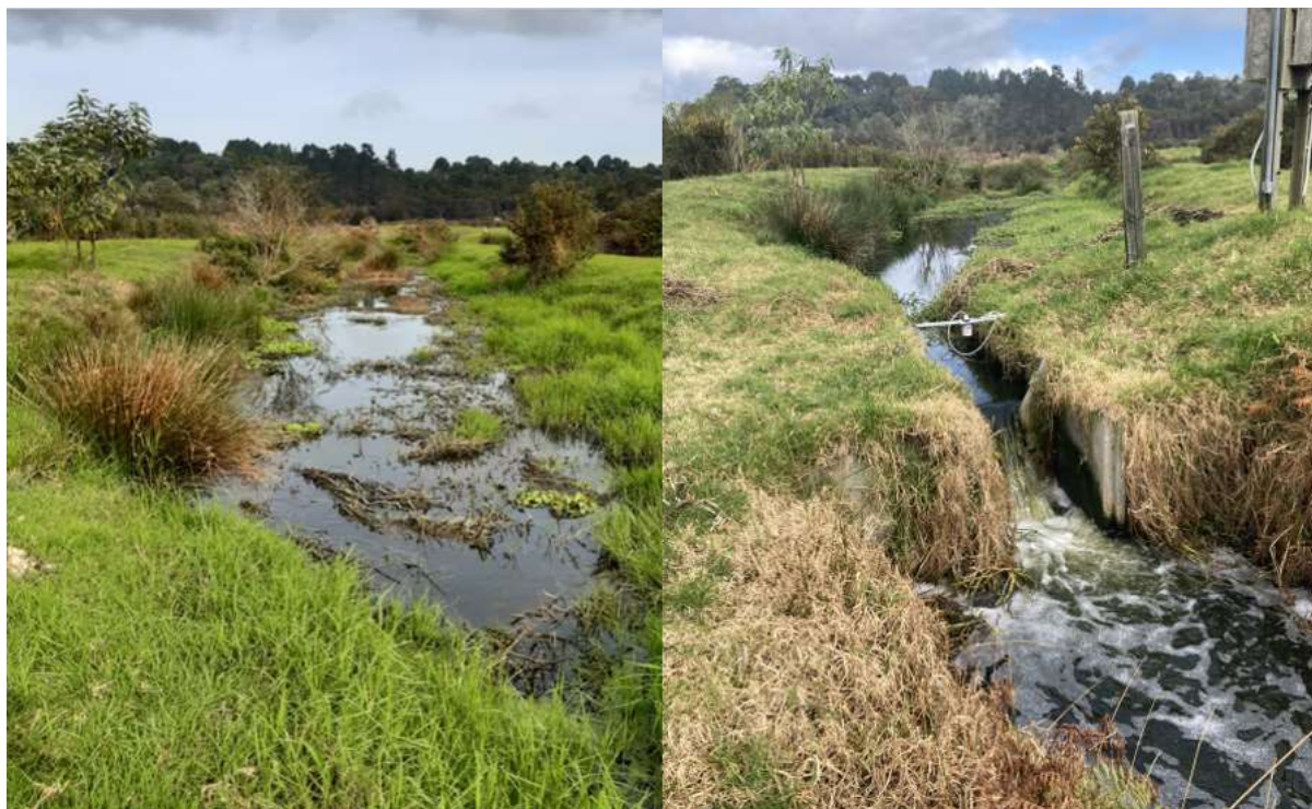
Figure 3-2 Constructed wetland system (left) and weir structure (right) located at the point of discharge at the Kaikohe WWTP. Image taken by report author 28/7/2021.
