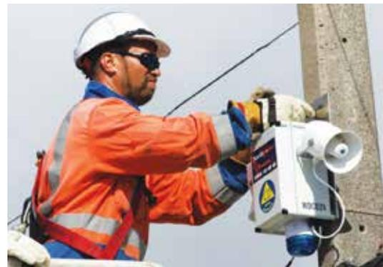
The tsunami siren network is tested twice a year at daylight savings weekend. Each daylight savings Sunday at 9.20am the siren network is tested by Civil Defence and Northpower/Top Energy and any maintenance issues are reported and corrected to keep the system in good working order.
